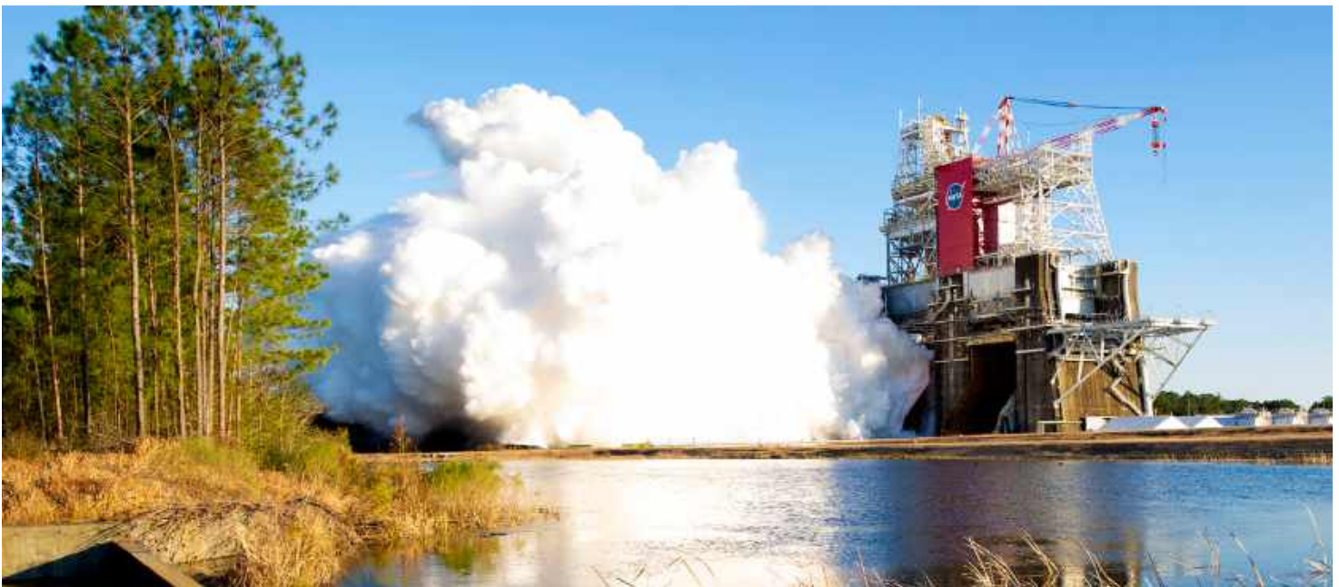
NASA Stennis provides unique facilities, such as the Thad Cochran Test Stand pictured here, for testing SLS RS-25 engines, controllers, and rocket stages.
